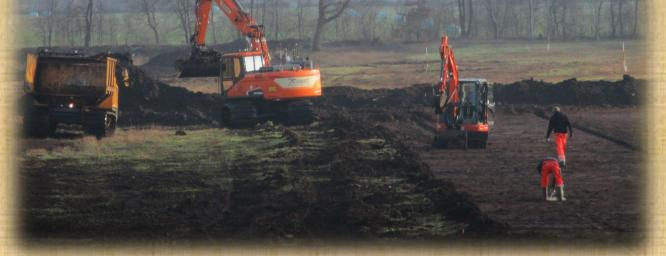
building of surrounding cables, bund, building of peripheral trench irrigation ditches (dividing and polder in 16 culture beds with width of 6 m), adjustable inflow and outlet
