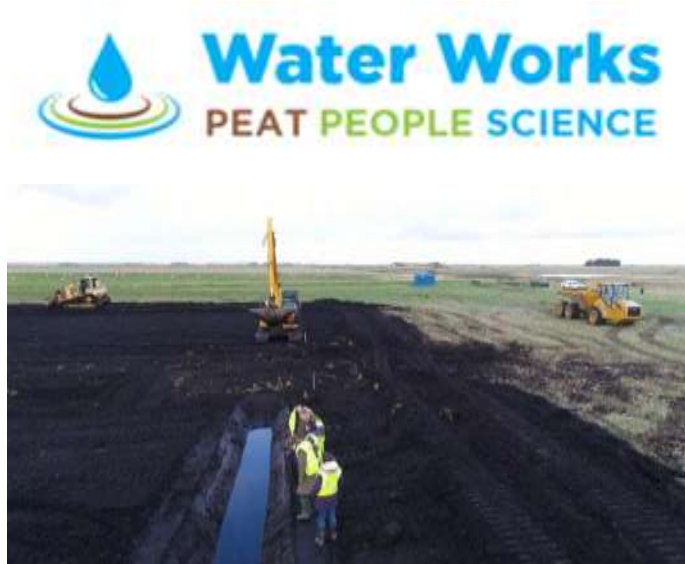
12 Ground preparation on site (Photo: Henry Stanier)
